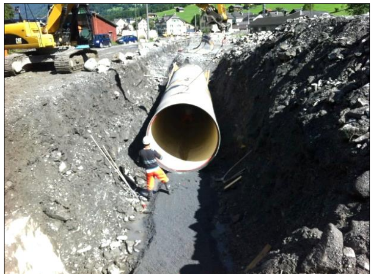
Installation DN 2200 made of fibreglass
