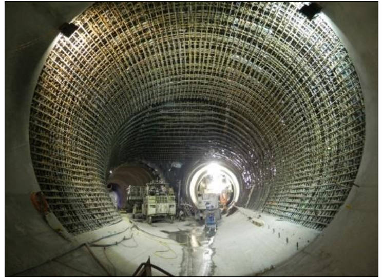
Upstream headrace concreted manifold Ø = 8.0 / 2 x 5.50 m
