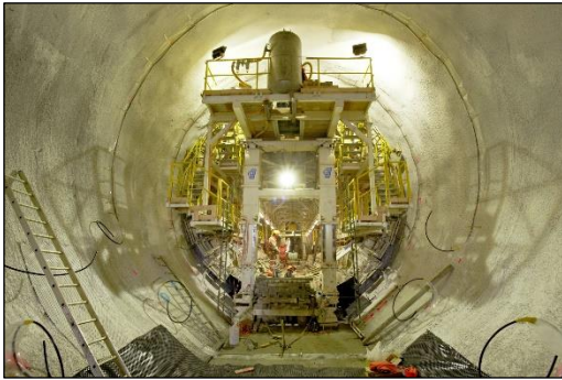
Headrace pressure tunnel formwork (Ø = 8.0 m)
