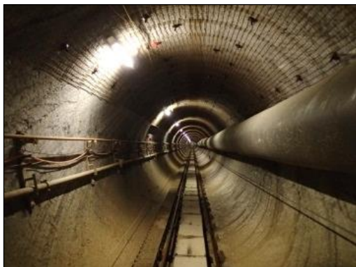
Excavated pressure shaft (Ø = 5.20 m, 85%)
