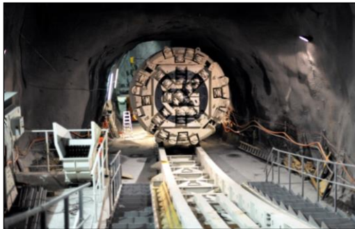
TBM Pressure shafts (Ø = 5.20 m, L = 1054 m)
