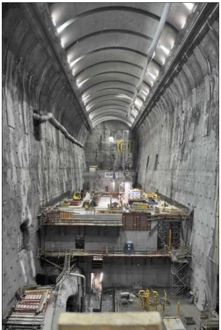
Excavated Powerhouse Cavern after starting of the first concrete works
