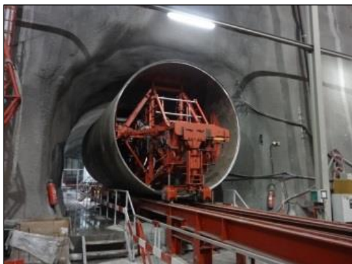
Steel lining erection of pressure shaft (Ø = 4.20 m)
