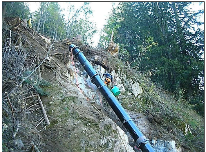
Installation of the cast iron penstock DN600 on the steep slope
