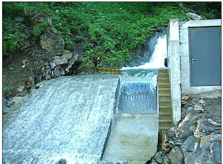
Fixed barrier with the Tyrolean system
