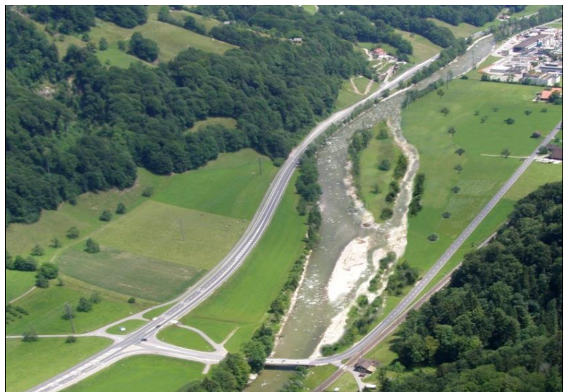
Side channel and intervention line - Langnau Widening, Werthenstein (composite photo)
