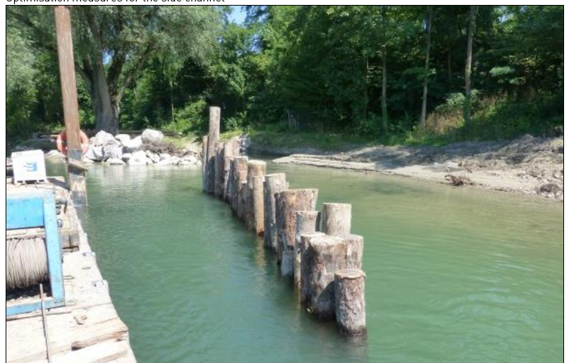
Stake barrier to optimise side channel flow (state of construction)
