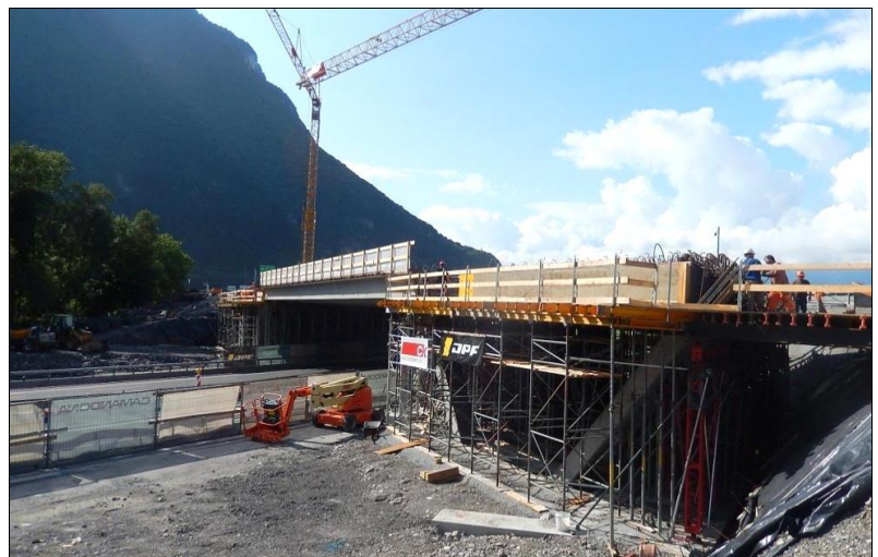
Installation of frame girder bridge – partly pre-fabricated
