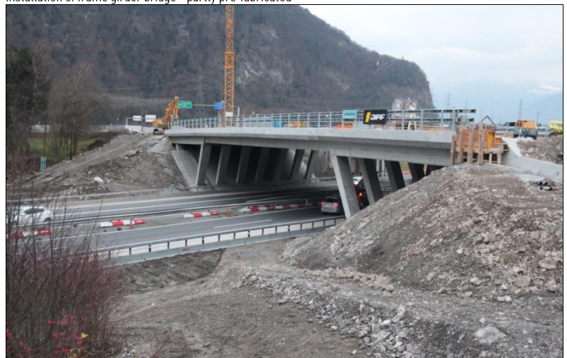
Completed structure after tightening of pre-stressed cables
