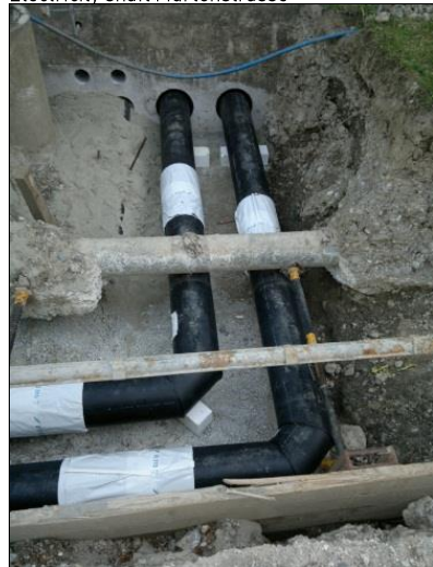
District heating pipes Murtenstrasse
