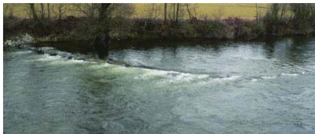
Figure 4. Upstream-facing micro groin at the Mur River in St. Michael/Upper Styria at low flow conditions (Photo courtesy of Otmar Grober).
