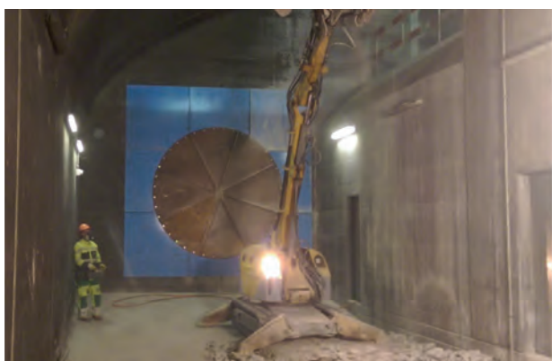
Figure 5: Demolition of ventilation units
