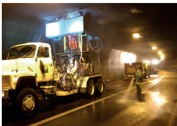
Figure 1: Sawing an exhaust air trap Figure
