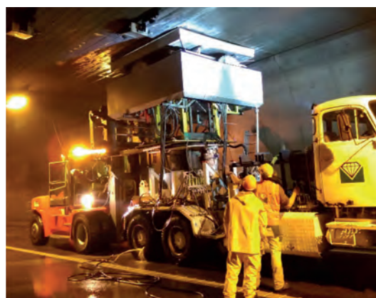
Figure 2: Removal of the sawn intermediate slab block
